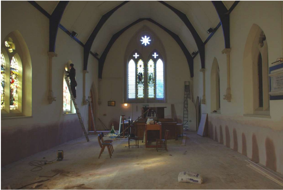
Reordering in progress, showing expanse of underfloor heating.
