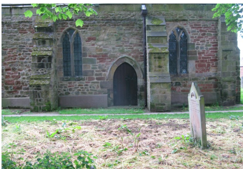
North wall before works
