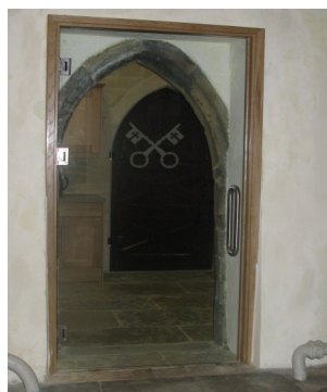
Glazed door to extension from nave
