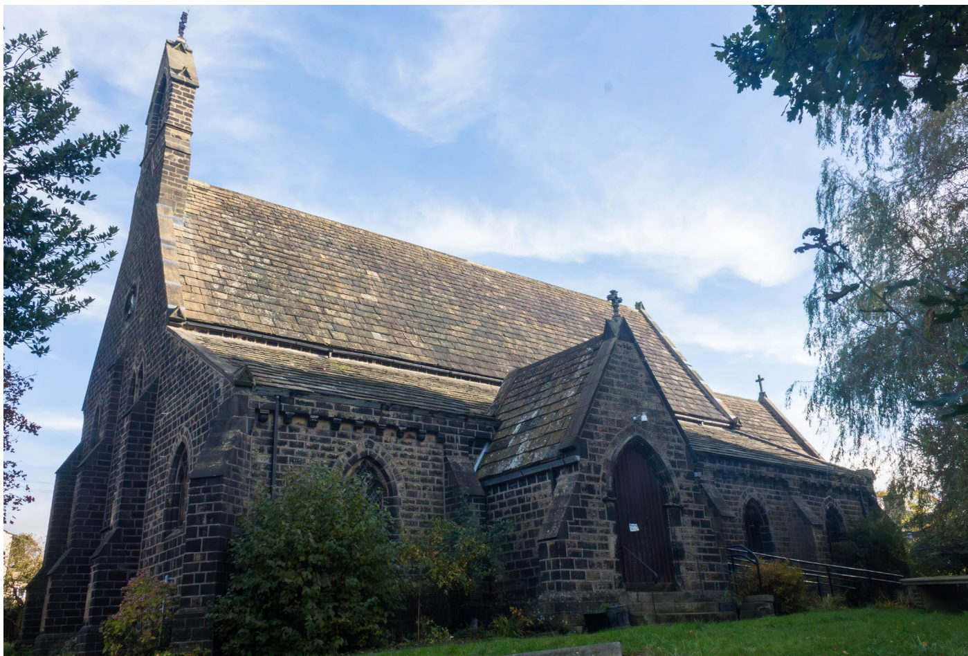
◀ ST LUKE'S PARISH CHURCH
