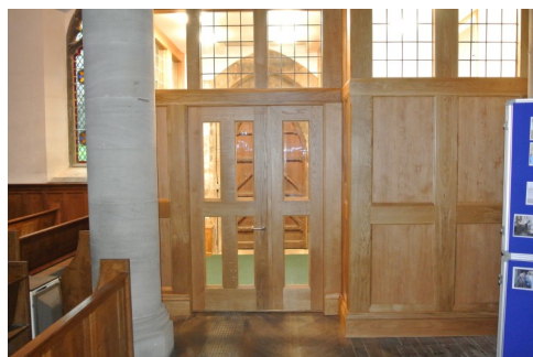
Draught lobby from nave
