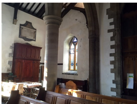
SW corner prior to works
